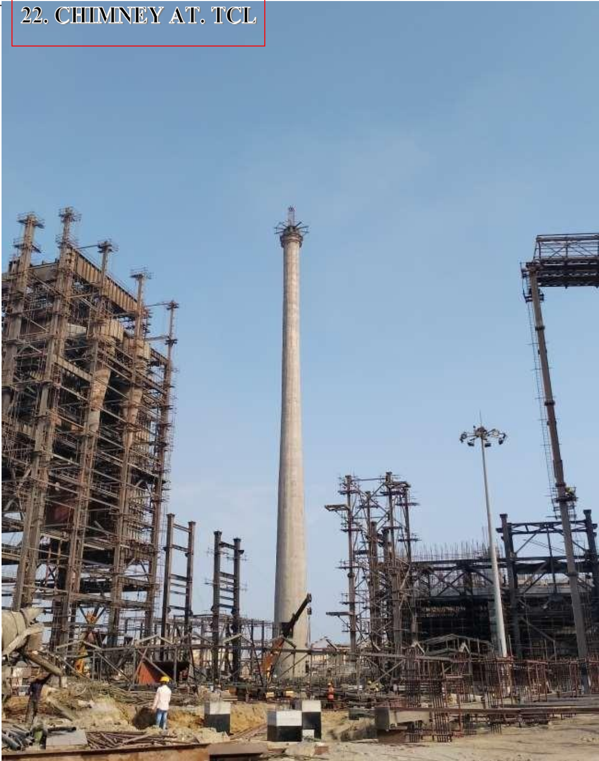
131 Mtr Ht. RCC Chimney At: Mithapur , Okha Clien:- Tata chemical ltd.
