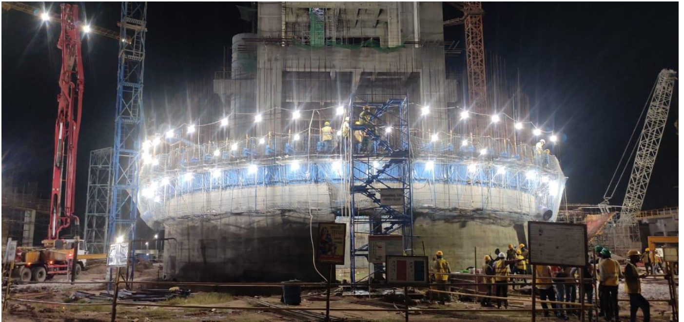
Bending Silo Erection at Ambuja cement Ltd. Nagaur (RJ)
